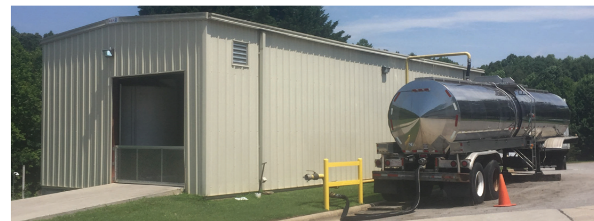
Reidsville Production Plant wastewater pre-treatment facility
